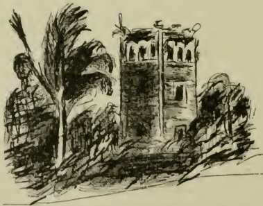
TOWER OF CHURCH OF ST. ANASTATIUS—Old Panama.
